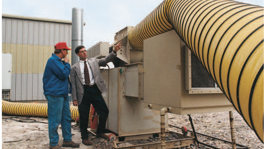
Polygon rental dehumidifiers controlled humidity for four months.
